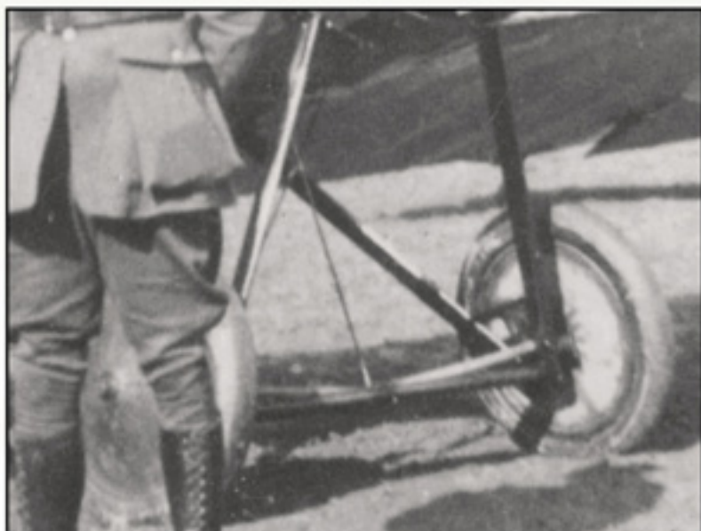
11 Undercarriage detail showing the usual angle of the split axles when absorbing the weight of the aircraft on the ground.
